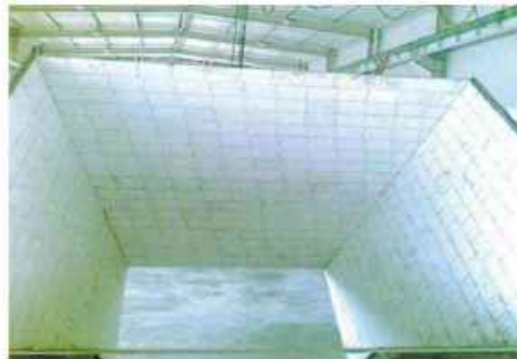
Ceramic Lined Silo
